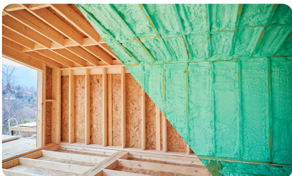
SPF insulation applied during residential wall framing
