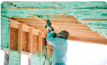
Exposed spray foam installed in residential attic space
